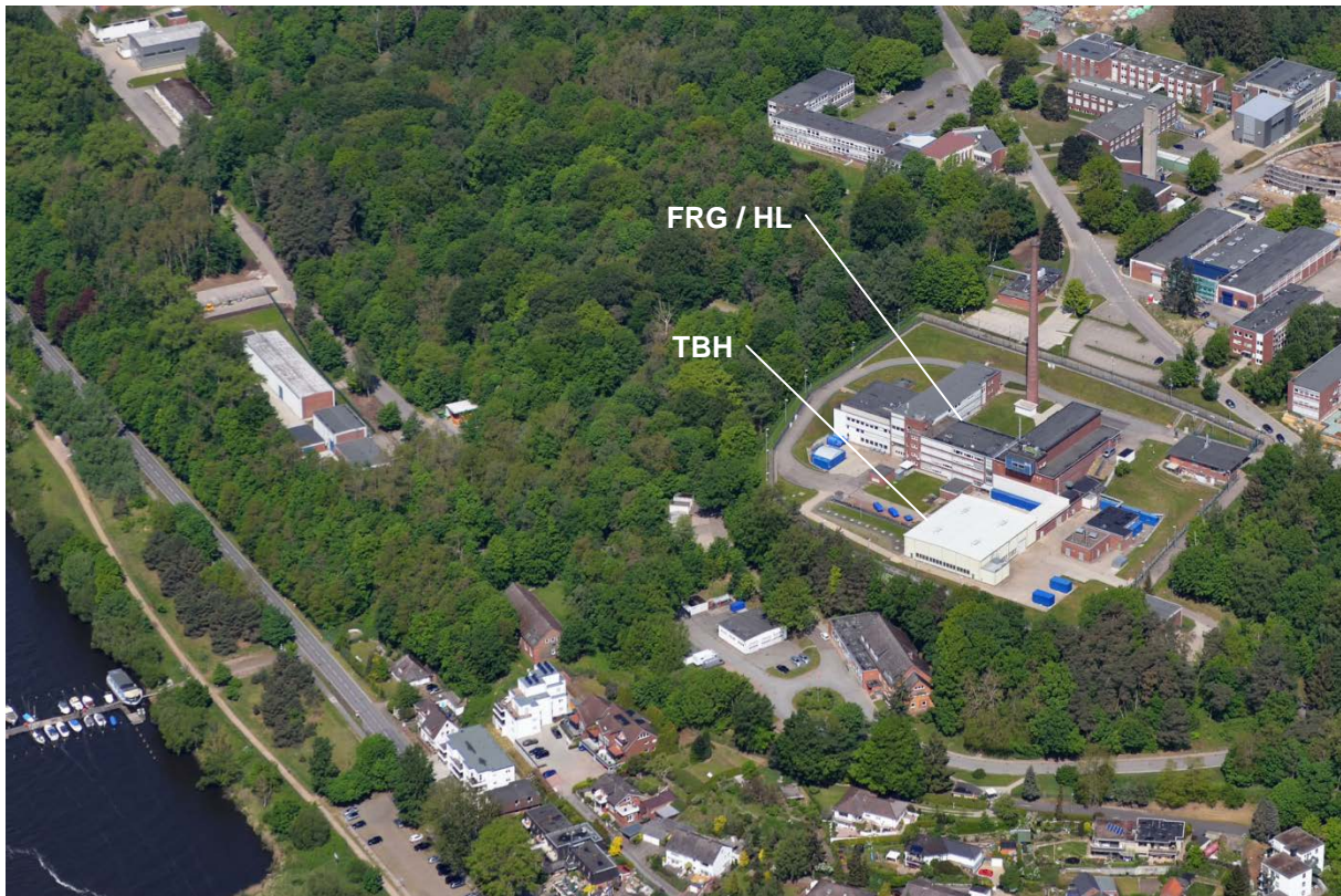
Figure 3-1: Aerial view of the TBH next to the FRG and the HL (from 2016)
